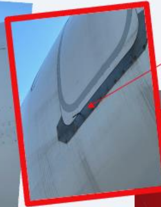
Damaged door seal
